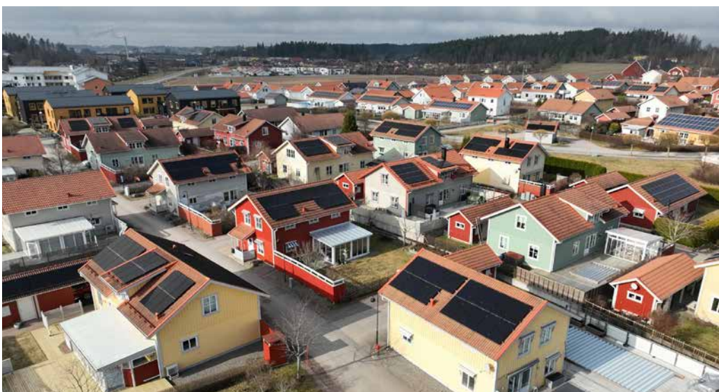
Since 2023, 500 homes in Gnesta, Sweden, have been equipped with Huawei's residential systems.
