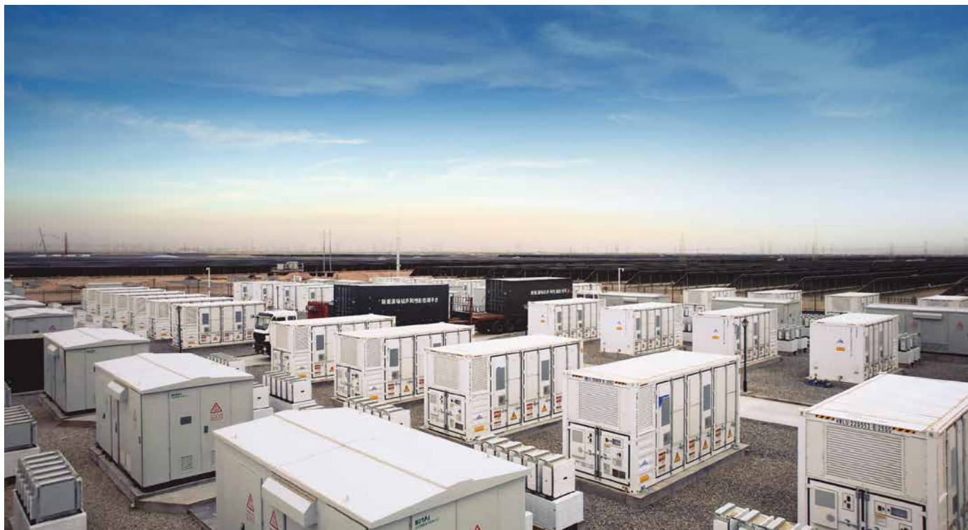
Huawei's 50 MW/100 MWh Smart String Grid-Forming ESS passed the grid-connection performance test in May 2024.
