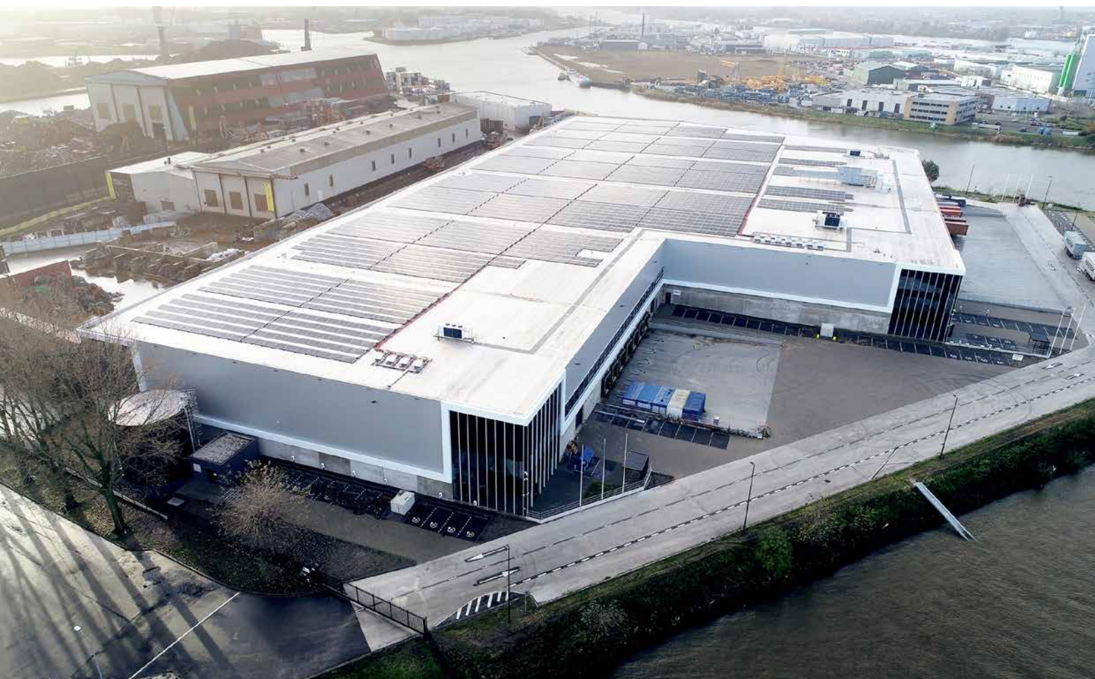
This rooftop installation in Dordrecht features 15 Huawei SUN2000-100KTL devices supporting a 2.7 MWp PV system.
