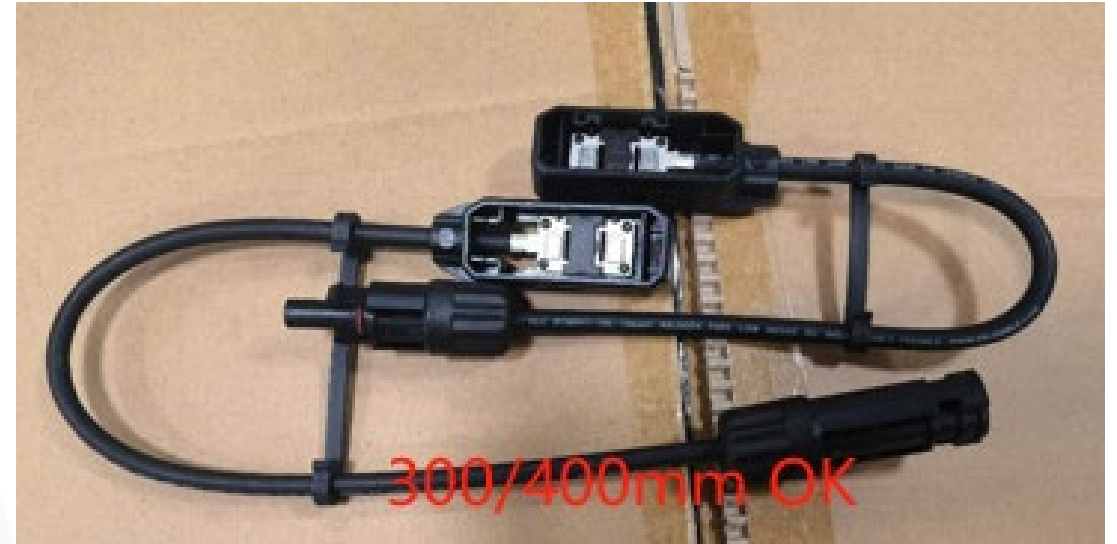
Correct junction box cable length of 300/400mm
