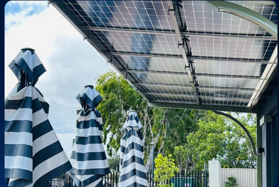
Sydney Display Center Solar Shade
