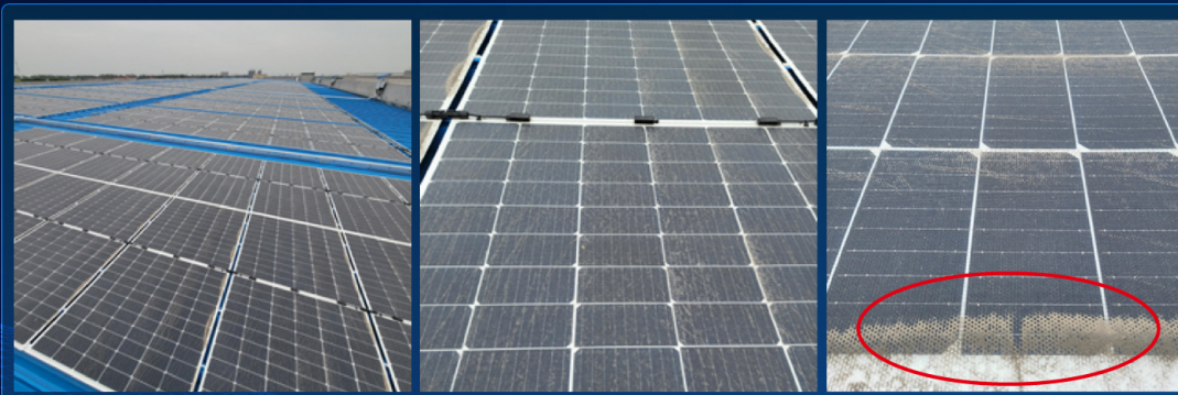
Deformation of polymer materials leads to dust accumulation
