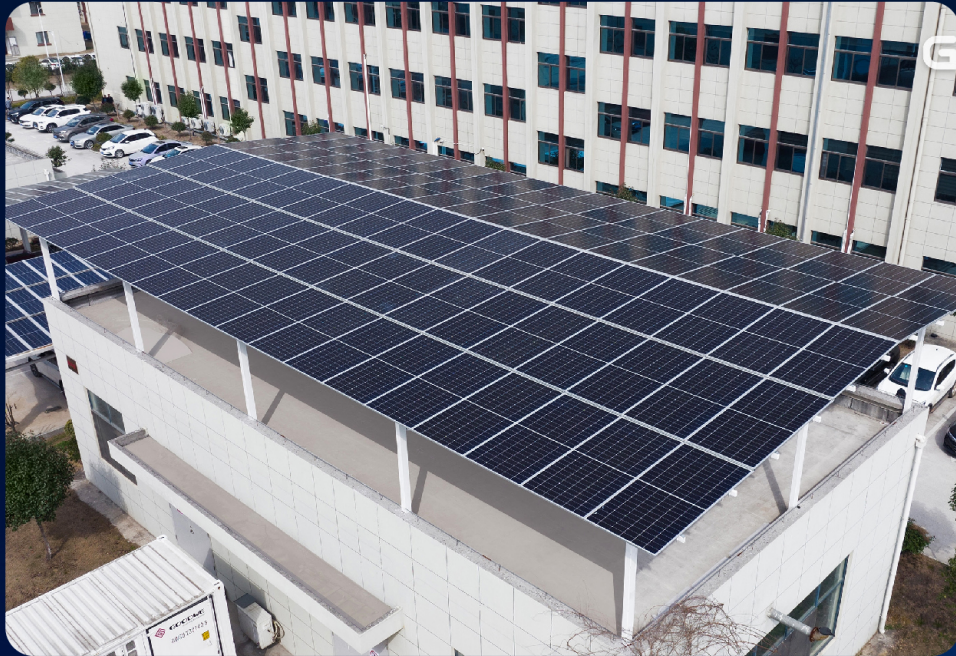
Guangde Production Base Solar Shed
