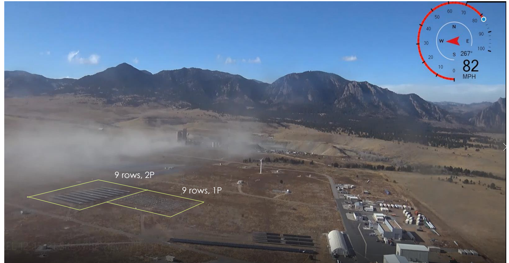
NREL Flat Irons Campus Installation
